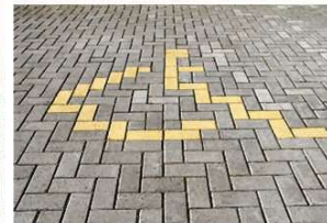
6. Disabled Parking demarcation
