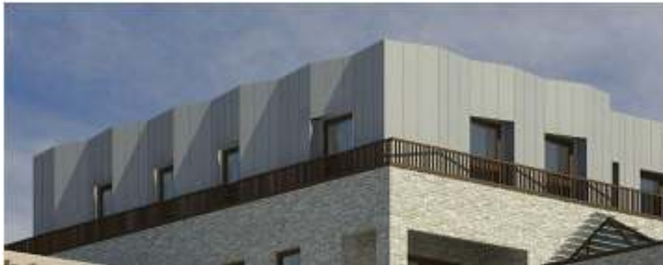
Fig 9 – lightweight materials on top floor of Principal Building
